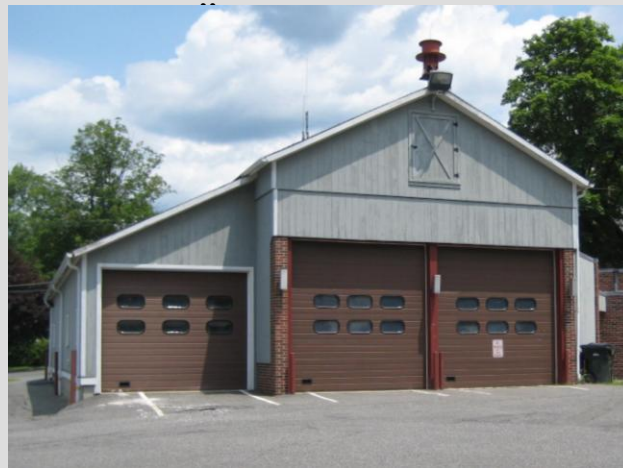
“Existing Apparatus Bays”
