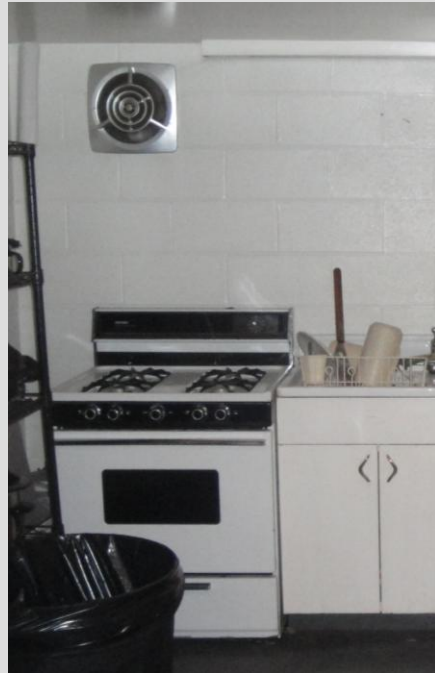
Non-Compliant Kitchen Exhaust System
