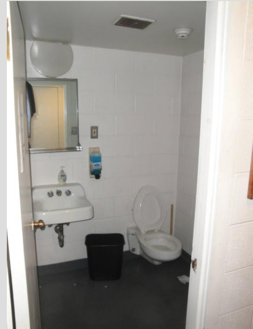
Building is Not Handicapped Accessible, Including Steps at Entry / Exits, Toilet Rooms and Split Level Building.
