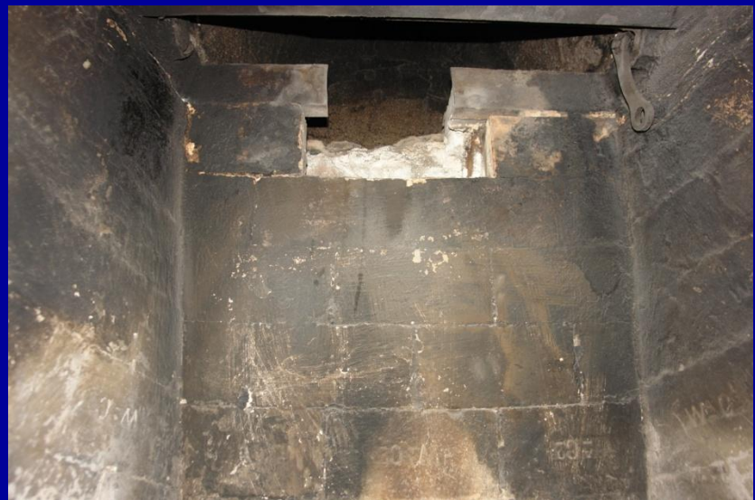
Damaged Damper
